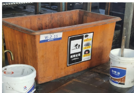
Tongtu Road Zero-Waste Plant
